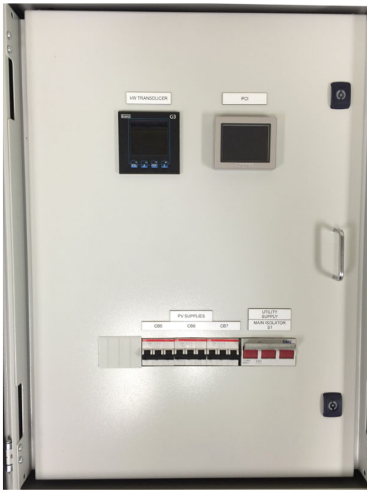
Zero Export, No Protection with KW transducer
